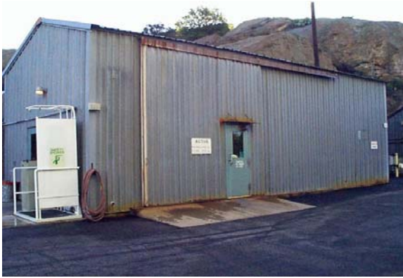
Figure A-5. Building 4044 Exterior
