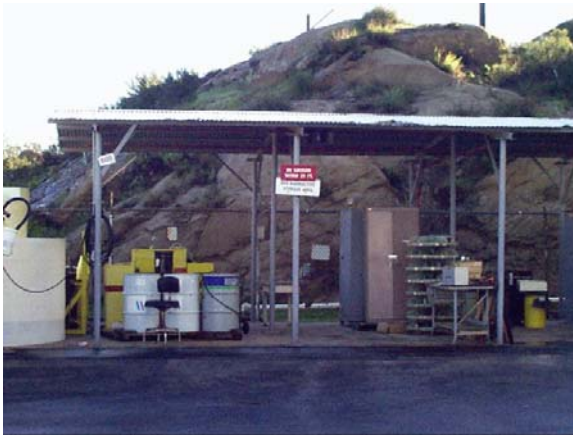
Figure A-7. Building 4688 Exterior
