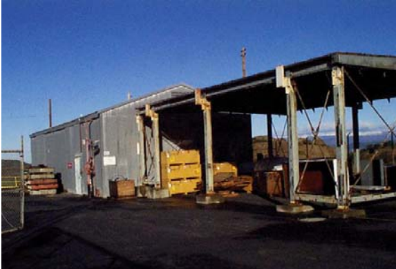
Figure A-4. Building 4075 and 4563 Exterior
