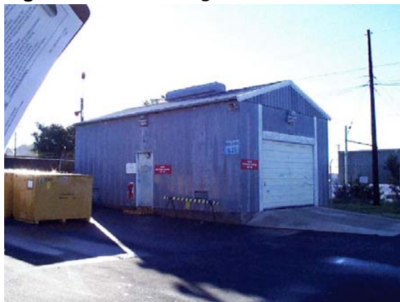
Figure A-3. Building 4621 Exterior
