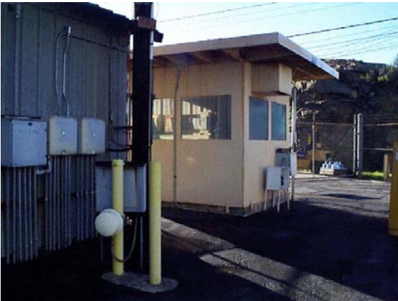
Figure A-9. Building 4658 Exterior
