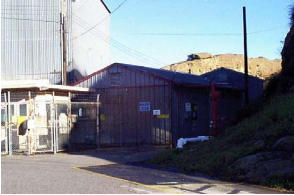
Figure A-8. Building 4034 Exterior
