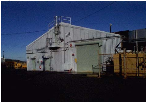
Figure A-1. Building 4021 Exterior
