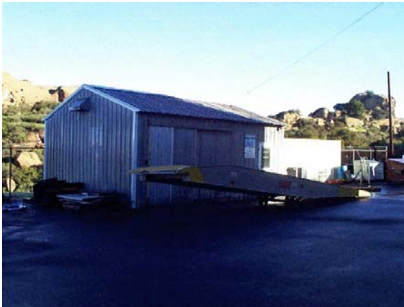
Figure A-6. Building 4665 Exterior
